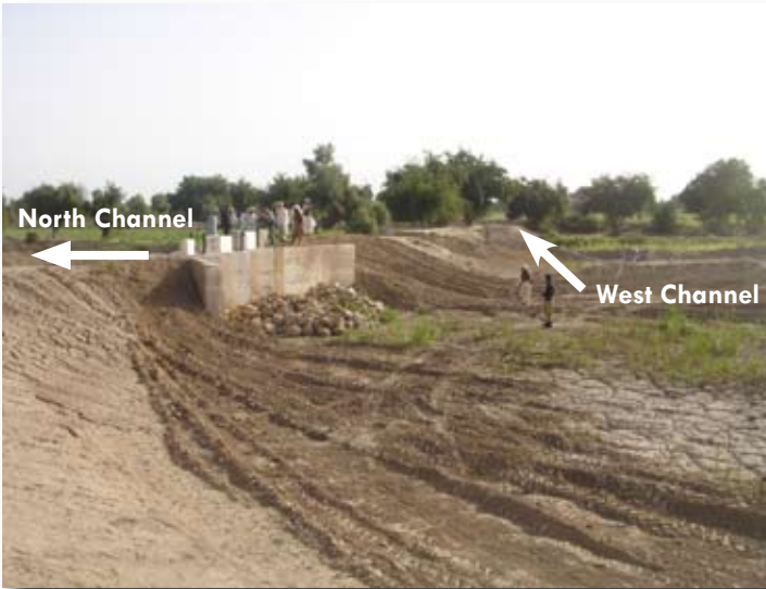
Figure 4. Solution: Flow division structure
