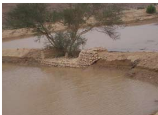
Figure 6 Stone reinforced overflow structure
