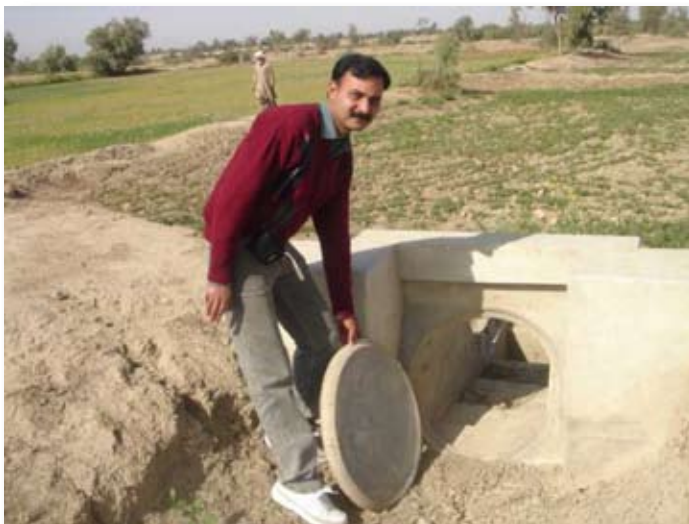
Figure 8 Improved field overflow structure
