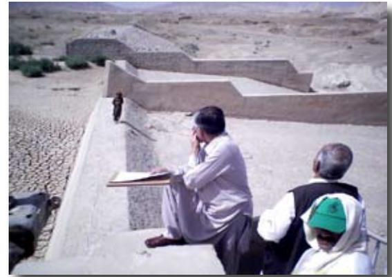
Figure 2. Weir structure, head regulator and canal at Shabo Headworks, Pishin district, Balochistan.
