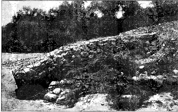
Figure 2 Example of insufficient side keying
