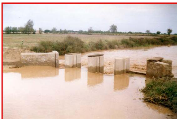
**Figure 5. Regulation and control structure for non-perennial Spate irrigation system (PARC)**
