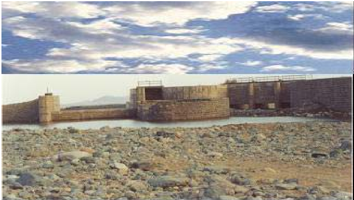
Figure 5: Undershot Wadi Laba diversion weir (Photo by Author 1 )
