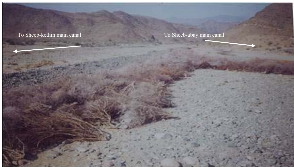
Figure 3: Traditional diversion structure, the jelwet (Photo by Author 1 )
