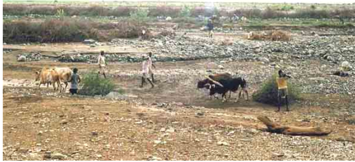
Repairing diversion spur Eritrea
