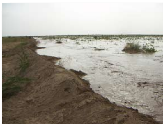
Figure 17 guiding water across huge fields with small field bunds, Gash, Sudan.
