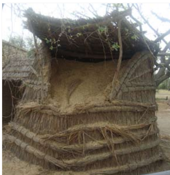
Figure 3. Pulla - local grain storage made of reeds and thatches. Grains are stored by cover of wheat straw, DG Khan, Pakistan
