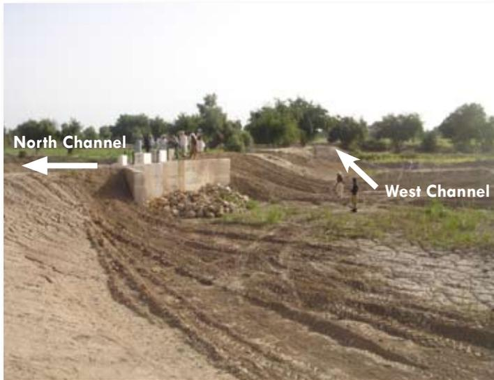
Figure 4. Solution: Flow division structure
