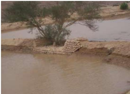
Figure 6. Stone reinforced overflow structure
