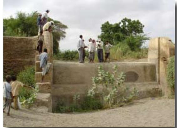
Figure 1. Drop structures to overcome level differences and dissipate energy: note the stepped construction
