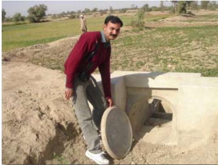
Figure 8. Improved field overflow structure
