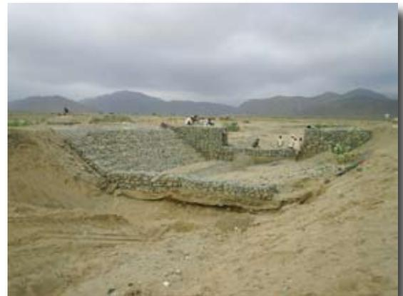
Figure 2. Flow division and channel bed stabilizer: important that apron has sufficient length
