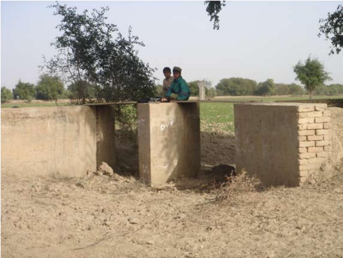
Figure 9. Intake gate with stop-logs
