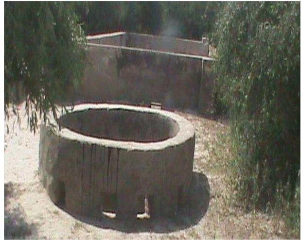
Figure 4: Reservoir with silting Basin - Dedh Village
