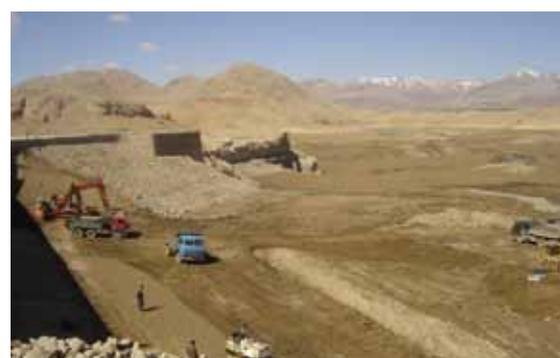
Figure 1: Repairing of a Bund Sultan in Ghazni province to collect spring water. Source (MEW 2006)
