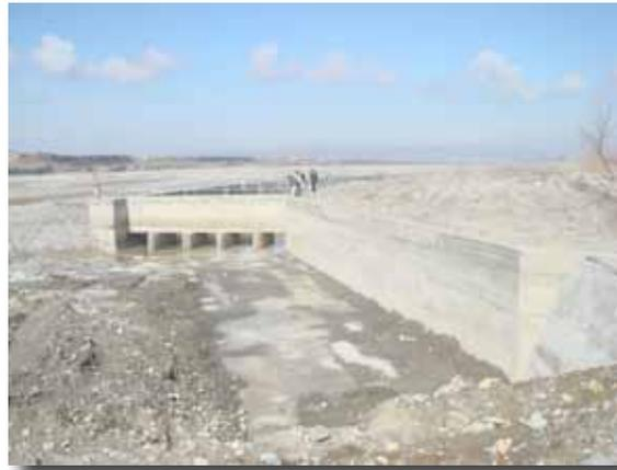
Fig 2: Bund and diversion structure in the Surkhrod ephemeral river and Amu basin area (MEW, 2012)
