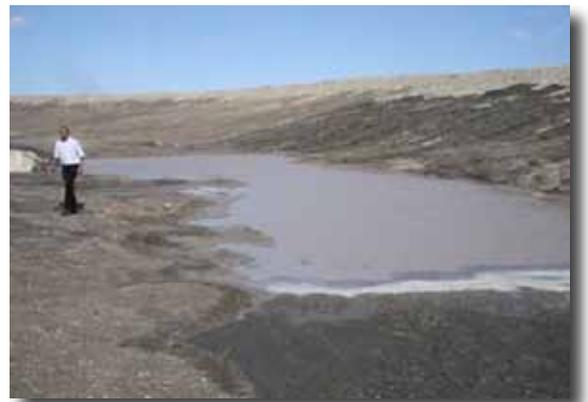
The photo shows a recently completed off stream reservoir, designed by and constructed under supervision of the writer, that will hold 120,000 m<sup>3</sup> of run-off mainly from a dry river bed and will be used to provide water for a 45 acre drip irrigation system. Due to the high cost of investment the farm will only produce high value crops mainly for export. In the picture the reservoir had just received some water from incident rains.
