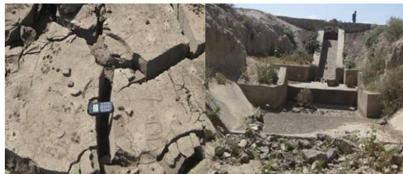
Figure 2: Sediments in the conveyance system of Boru Dodota Spate Irrigation Schemes
