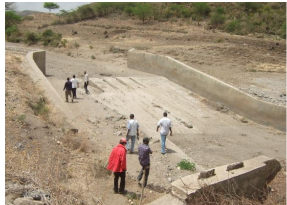
Figure 5: Site visit (Headwork at Bililo Small Scale Spate Irrigation)
